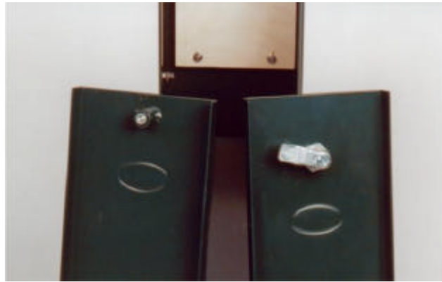
R150 covers – screw and cam-lock fixings
